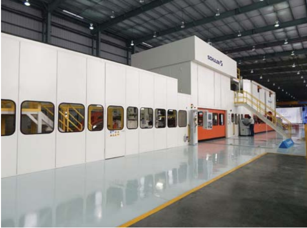
Within just seven weeks, Schuler modernized transfer and blank loader of Ford's large panel press in Cologne.
